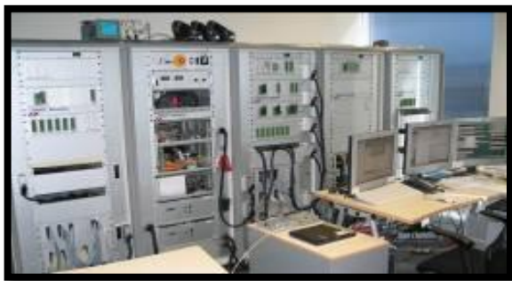
Figure 7: MBtech HiL test center operation for control units and networks
